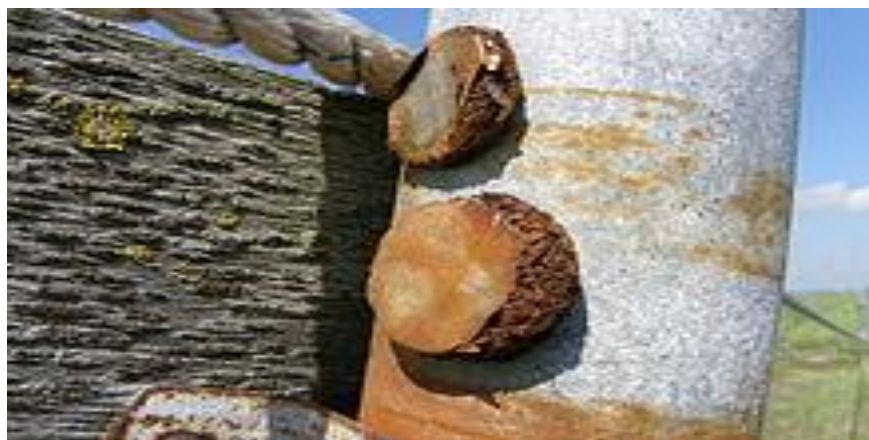
Fig.2 These neodymium magnets corroded severely after 5 months of weather exposure
