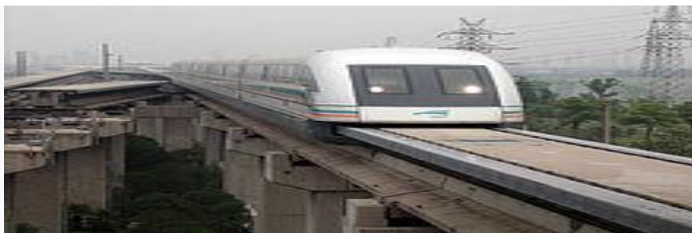
Fig.12 The Trans rapid system uses servomechanisms to pull the train up from underneath the track and maintains a constant gap while travelling at high speed
